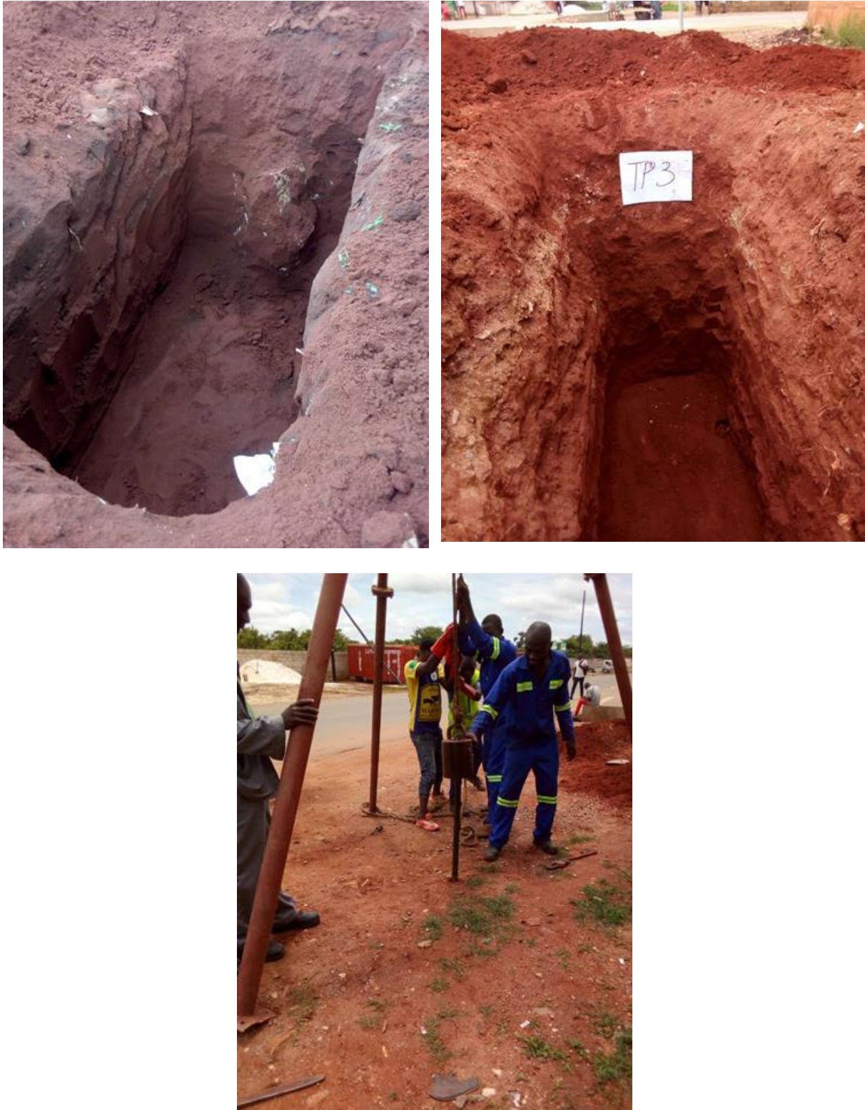
Figure 2: Chainda Trial Pits and Dynamic Cone Penetration (DCP) Test
