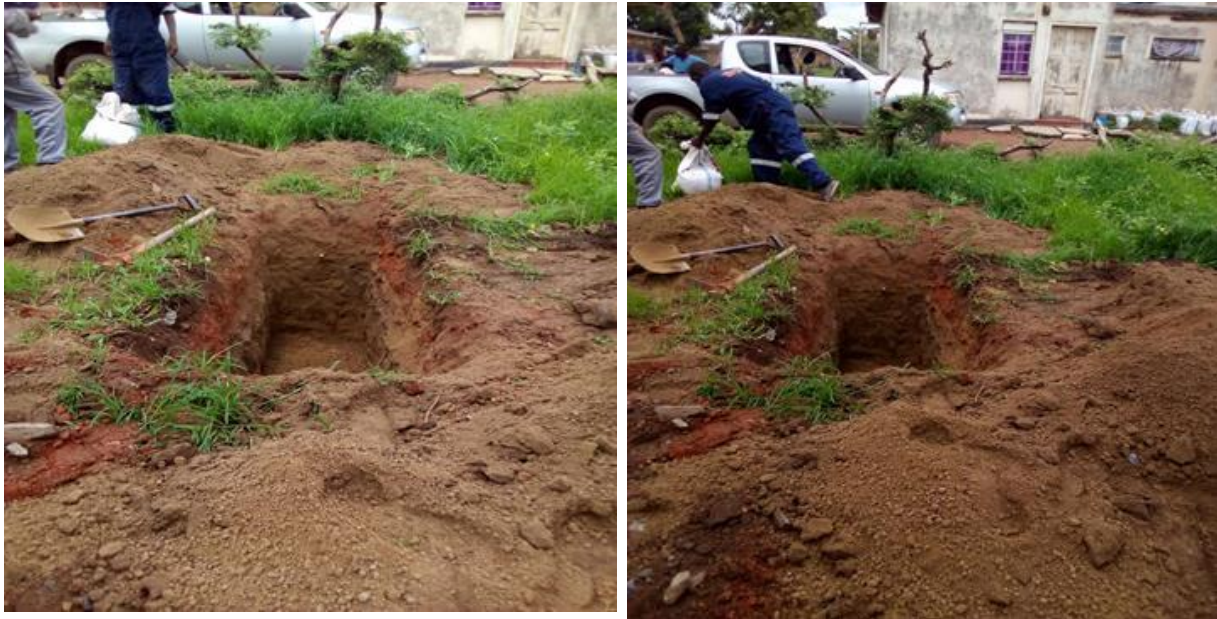
Figure 4: Kamanga (Nkoloma) Trial Pits
