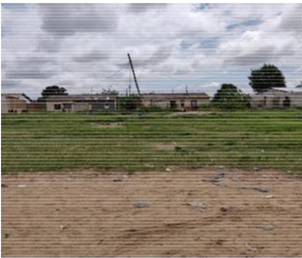
Figure 23: Pole Tilted Due to Weak Founding Soils near Mutamba Grounds
