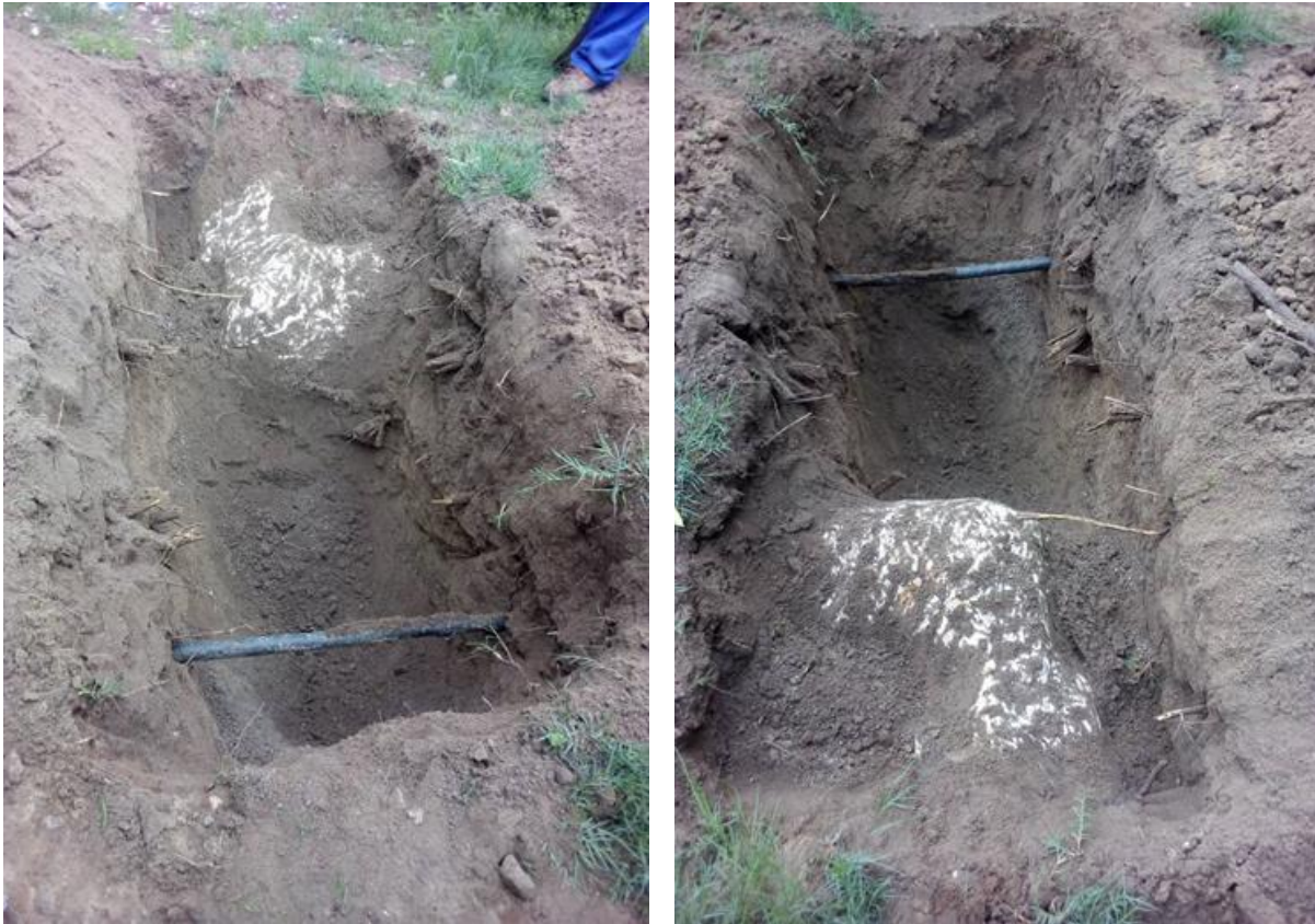
Figure 6: Chawama Trial Pits
