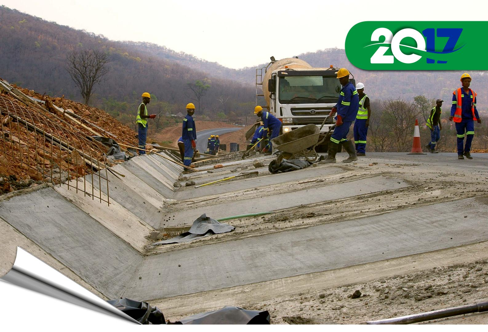
Rehabilitation of the Great East Road Project – ZM/FED/022-409 Construction of concrete-lined drains between Luangwa Bridge and Nyimba, Eastern Province. These are important for preventing rain water from penetrating the substructure of the road hence weakening the road.
